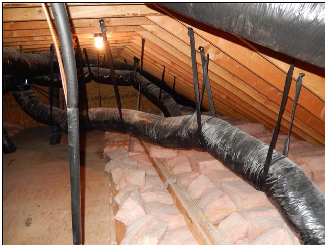
8.0 Item 1(Picture) Attic insulation
