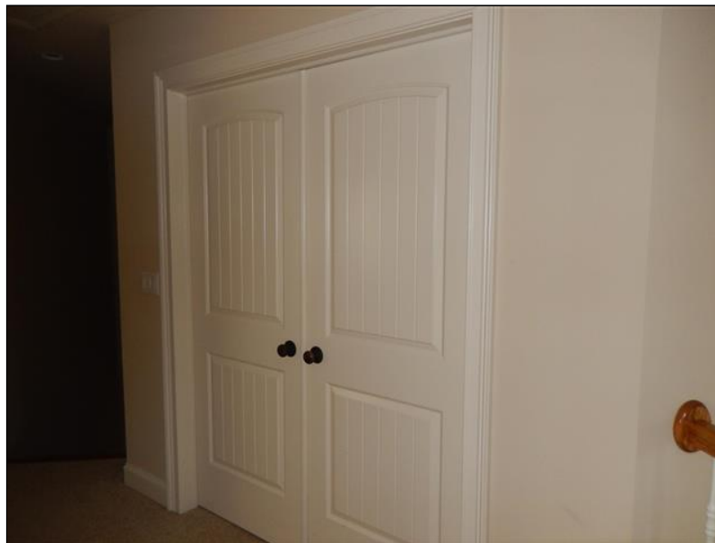
9.5 Item 2(Picture) Master bedroom door
