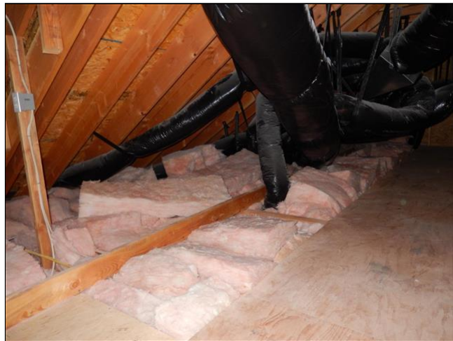
4.3 Item 4(Picture) 2nd floor duct work
