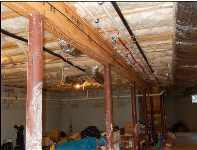
3.2 Item 1(Picture) Steel columns
