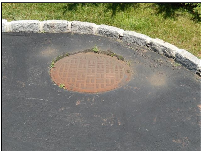
2.2 Item 1(Picture) Driveway manhole
