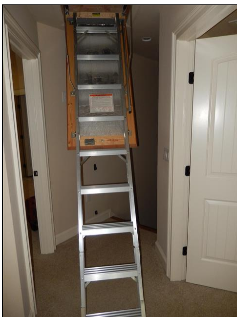
1.4 Item 3(Picture) Attic stairs
