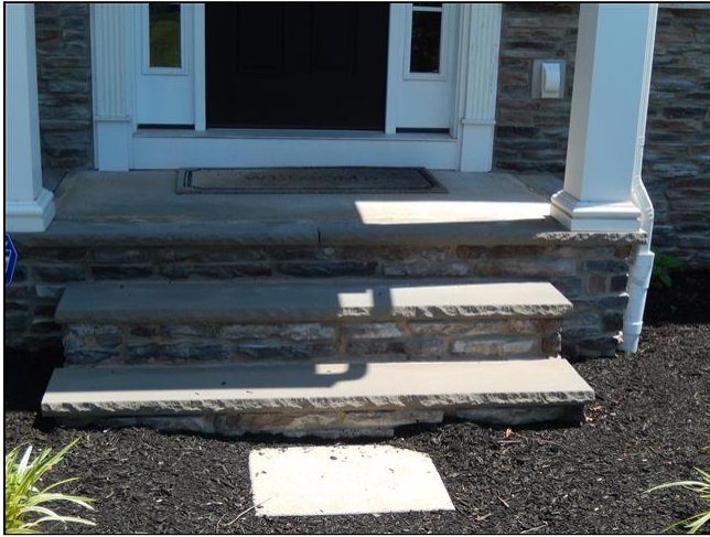
2.3 Item 1(Picture) Front stoop
