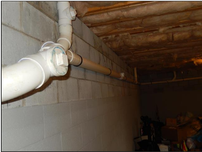
5.4 Item 1(Picture) Main waste pipe
