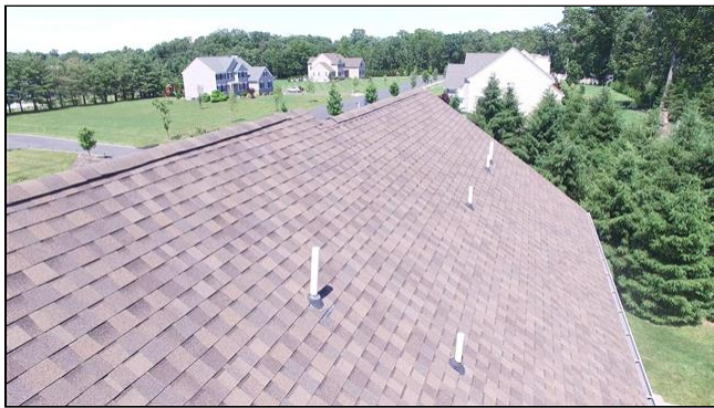
1.0 Item 1(Picture) Shingles
