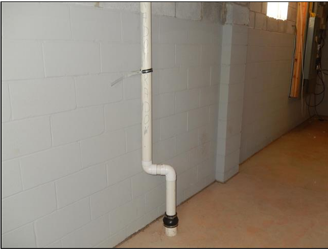
3.1 Item 1(Picture) Block wall
