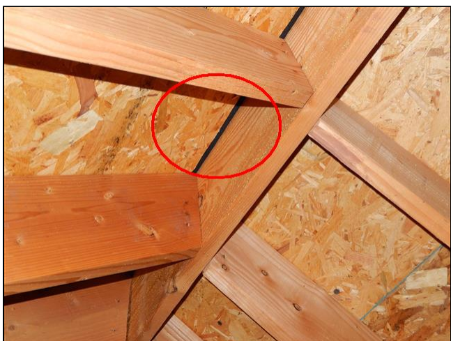
8.3 Item 1(Picture) Ridge vent
