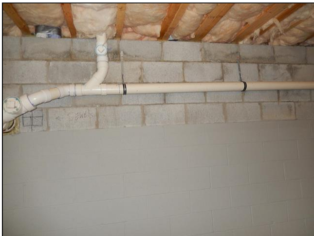
3.0 Item 1(Picture) Block foundation walls
