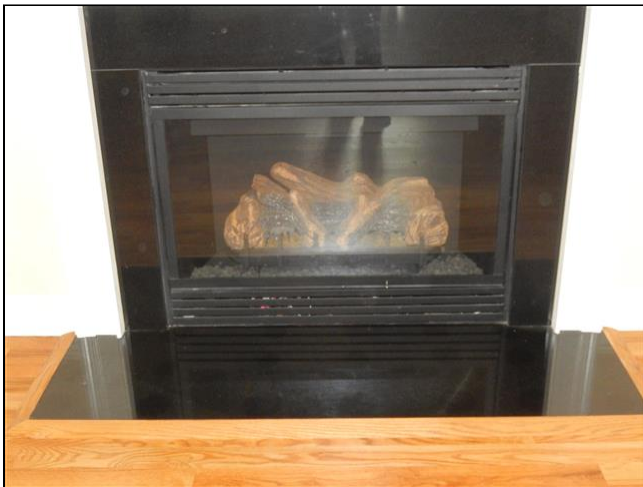
7.0 Item 1(Picture) Gas log fireplace
