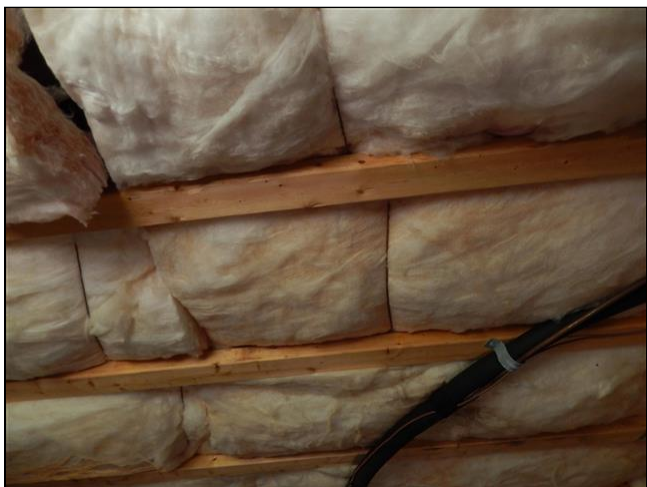
8.1 Item 1(Picture) Floor insulation
