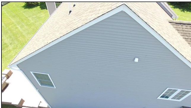
2.0 Item 1(Picture) Siding
