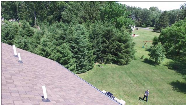
1.3 Item 1(Picture) Roof penetrations
