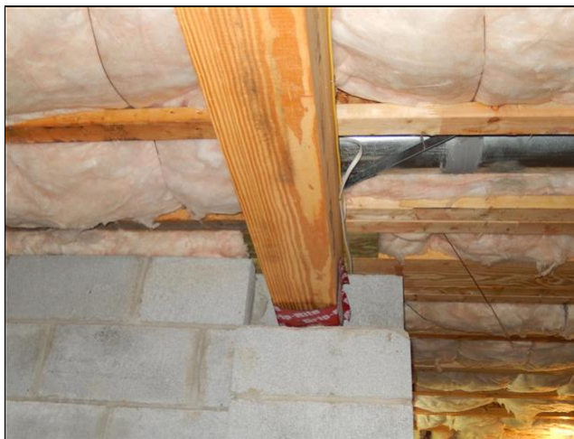
3.4 Item 2(Picture) Main beam
