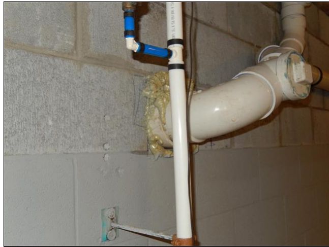
5.4 Item 2(Picture) Main waste pipe
