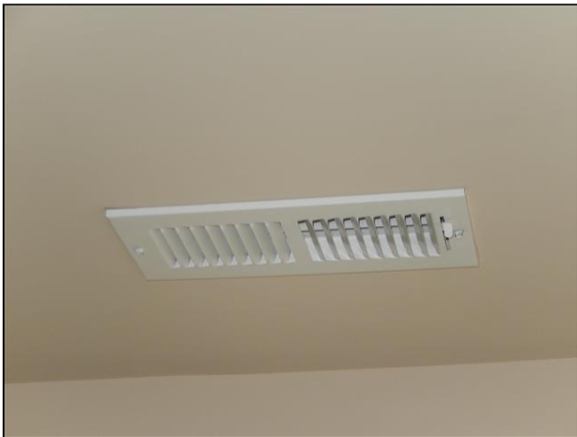
4.8 Item 3(Picture) Ceiling register - typical
