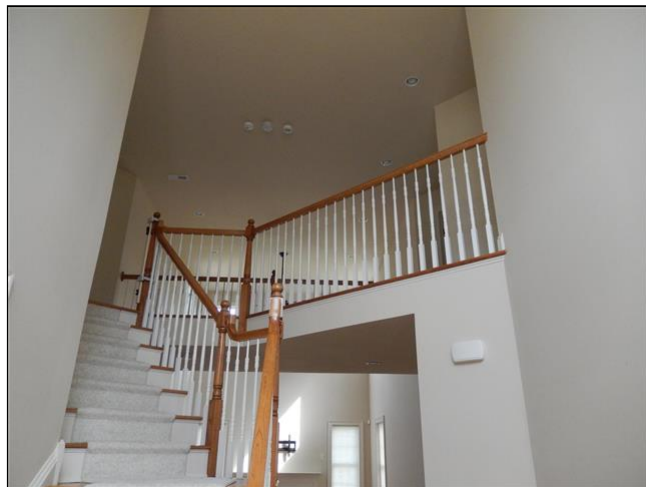
9.3 Item 2(Picture) Stairs to upstairs landing
