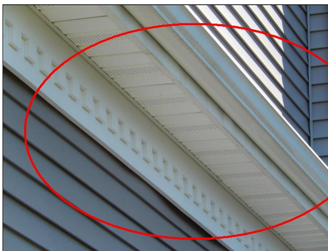
8.3 Item 2(Picture) Soffit vent
