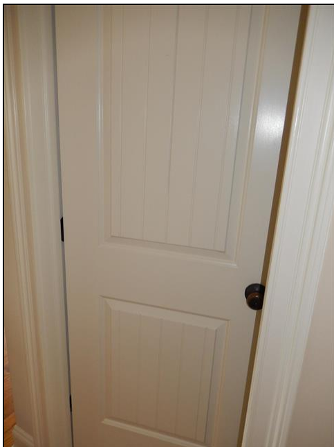
9.5 Item 1(Picture) Interior door - typical
