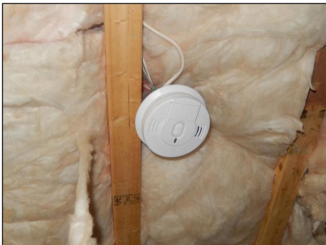
3.4 Item 1(Picture) Ceiling joist
