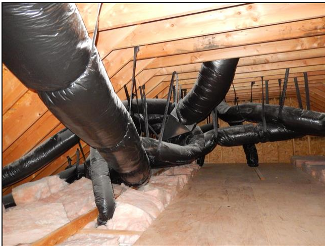
4.3 Item 3(Picture) 2nd floor duct work
