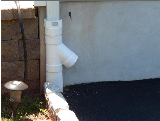
1.1 Item 1(Picture) Downspout discharge
