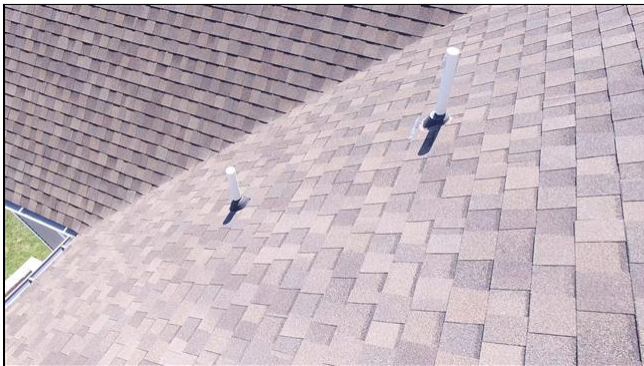
1.2 Item 1(Picture) Roof penetrations
