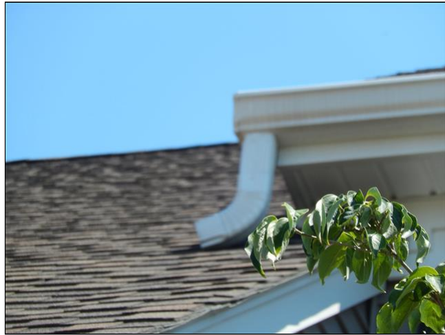
1.1 Item 2(Picture) Upper gutter discharge
